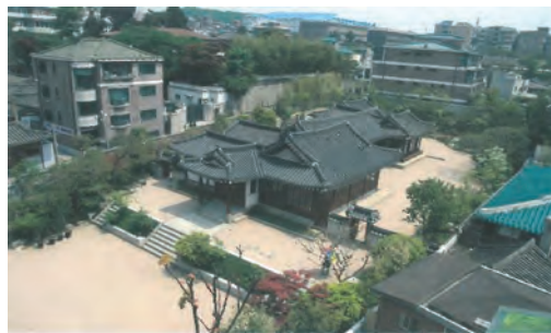
(a) Aerial view
